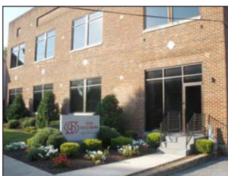
GALAXY CONTROL SYSTEMS CORPORATE HEADQUARTERS WALKERSVILLE, MD
