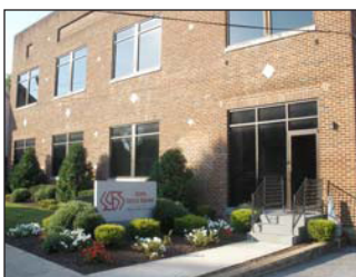
GALAXY CONTROL SYSTEMS CORPORATE HEADQUARTERS WALKERSVILLE, MD
